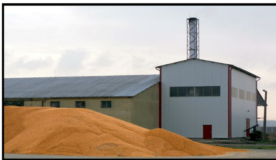
Picture 4 The broiler after reconstruction view
